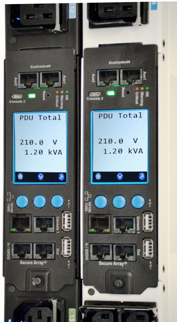
Figure 3: Remote power monitoring captures data that can be used in DCIM to trend power use, estimate remaining capacity, adjust for underutilized equipment and ensure failover.
