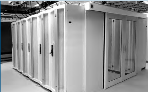
Figure 9: Aisle containment doors are available in various styles and widths. Ensure a good seal between the door frame and the sides of the adjoining cabinets. Consider a door that includes a mechanism to return and maintain it in a closed position.
